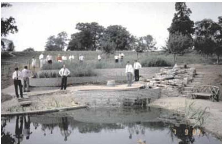
Pic. 1: The Oaklands Park system in its first year of operation showing the newly-planted stages down the hillside being inspected by the UK coordinating group.
