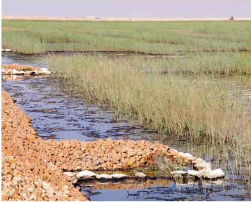
Plate 2: Inlet structure of one of the 24 ten-hectare surface flow wetland cells.
