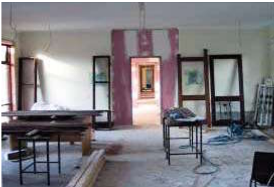
Meeting Rooms of the CSL, during refurbishment
