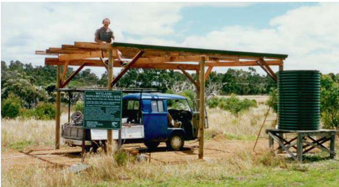
Construction of the Wetlands Education Centre, Denmark, in 1996.
