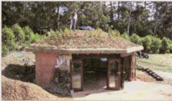
German volunteer architecture student Steffen Schulz checks the garden roof on the Sanctuary building with its native garden roof.
