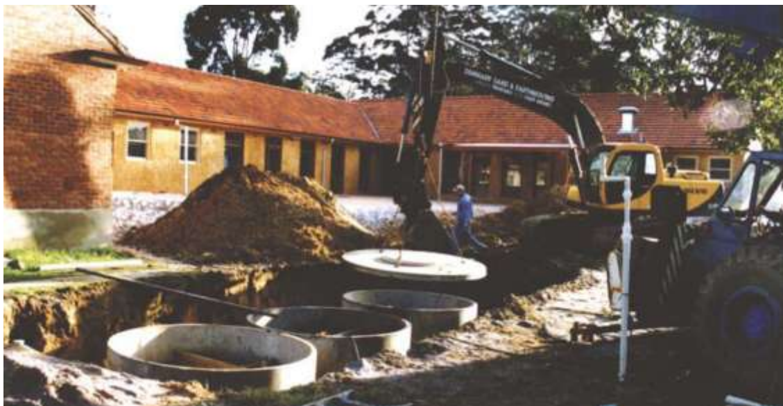
BioMAX wastewater recycling system at the CSL in 2004
