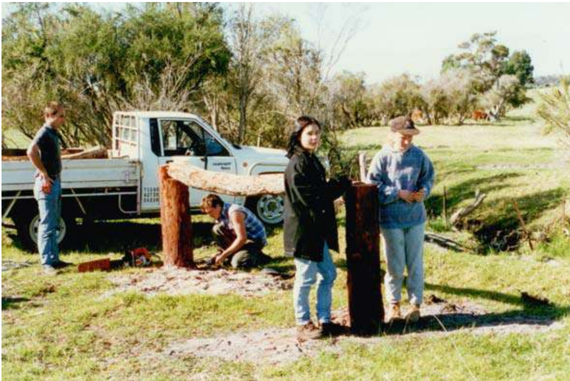
LEAP participants constructing fencing along a riverbank, Albany, 1996
