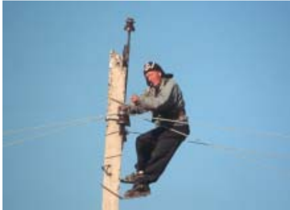
Removal of the deadly power lines at Lake Tengiz in Kazakhstan.
